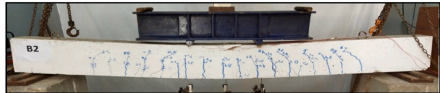
(b) Crack Patterns for the Tested Beam B2
